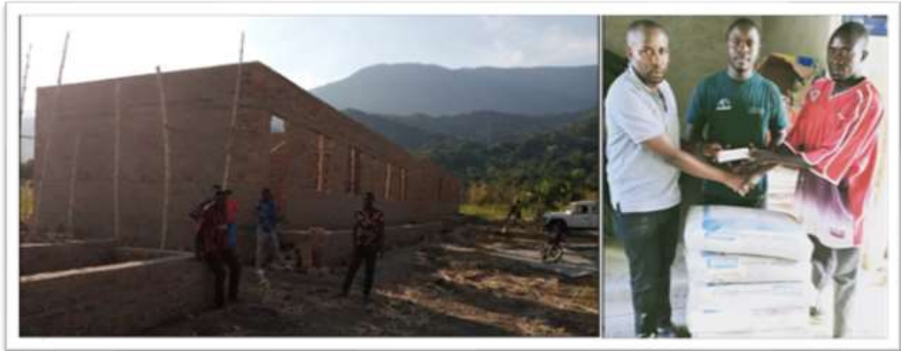
Figure 5: Constructed Ikule Secondary School (left) and USNFR officers handing over cement bags to Ikule Village Chairman (right).
